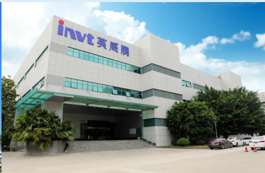
Shenzhen Fuyong Industrial Park
