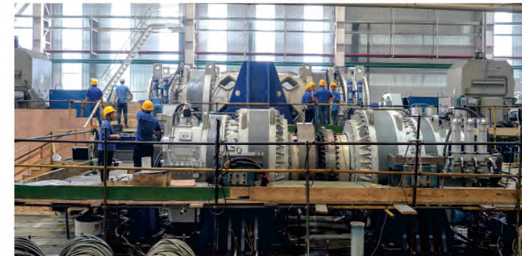
16MW+6.5MW试验台 Test Bench(16MW+6.5MW)
